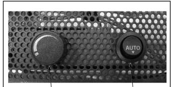
Blower Speed Control Knob (rheostat) Manual / Auto Rocker Switch
